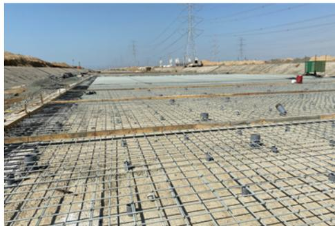
11,000 kilometers of GFRP rebar reinforce a concrete flood mitigation channel in Jizan, Saudi Arabia, and enable its 100-year service life. Source: Mateenbar
